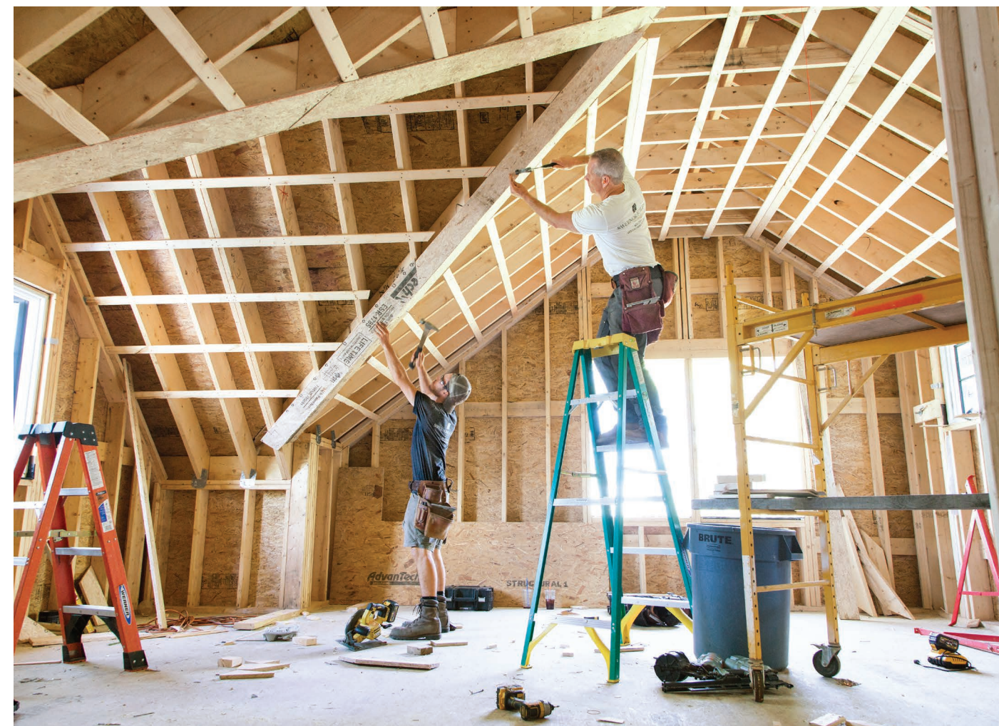
ABOVE: Contractor Jeff Sweenor (on ladder) and his son, Ryan, frame the vaulted ceiling in the second story above the freestanding garage, creating a dramatic space for a future guest suite.
