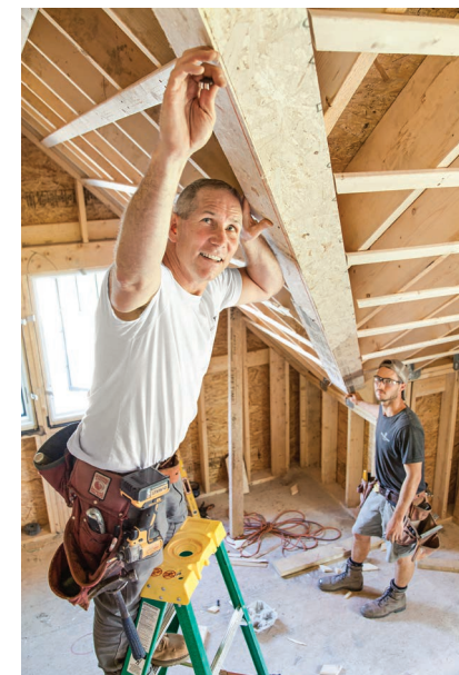
ABOVE: Contractor Jeff Sweenor (on ladder) and his son, Ryan, frame the vaulted ceiling in the second story above the freestanding garage, creating a dramatic space for a future guest suite.
