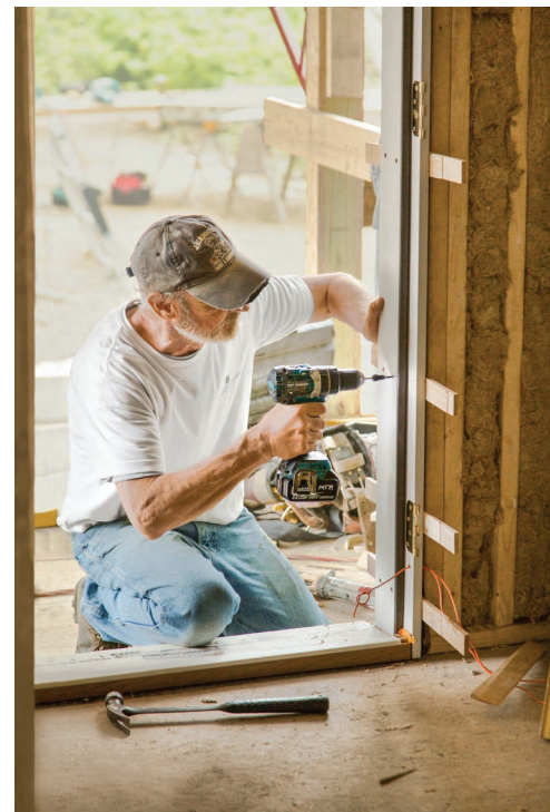
LEFT: Mike Rich trims out a doorway with moisture-resistant radiata pine.
