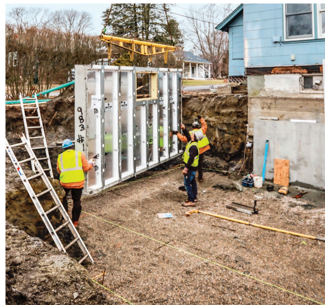
BOTTOM RIGHT: Tom Silva and Jeff Sweenor, the builder on the Jamestown project, check the measurement for the step-down addition's foundation height.
