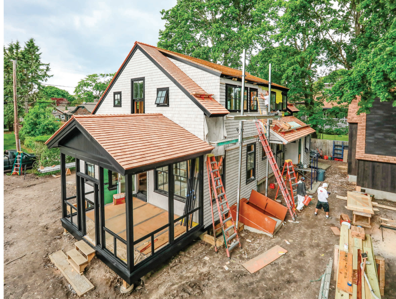
ABOVE: Red cedar roof shingles and white cedar sidewall shingles with woven corners (meaning no corner boards) are hallmarks of coastal New England cottages. Unadorned, flat exterior trim on rake boards, windows, and doors completes the look.
