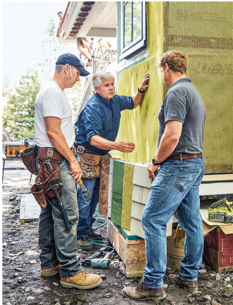
ABOVE: Tom Silva and Kevin O'Connor discuss a vinyl-mesh wall wrap with builder Jeff Sweenor. The mesh helps the white cedar shingles dry from the back side, increasing their life span and keeping moisture out of the house.
