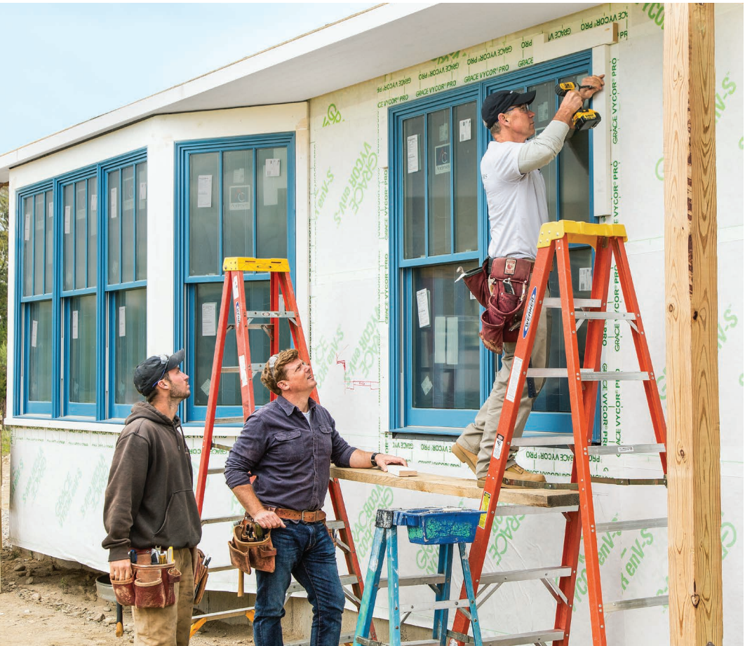
TOP: The wood-look capped-polymer porch deck will be impervious to water damage. LEFT: Contractor Jeff Sweenor trims out one of the hurricane-rated, aluminum-clad wood windows as his son, Ryan, an apprentice on the job, stands ready to assist. TOH TV host Kevin O'Connor dropped by to check out the house's progress. ABOVE: Ryan Sweenor readies a preprimed radiata pine trim board for installation.
